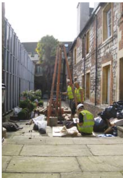
Trial pits and bore holes being dug outside the library
