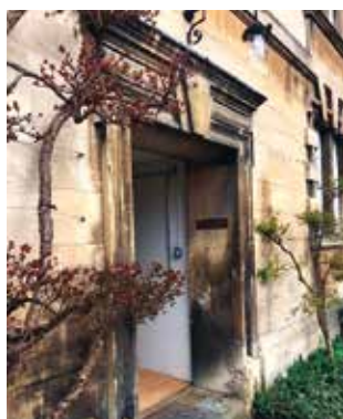
Entrance to V staircase
